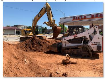
made to remove four tanks and investigate the proper closure of the other two tanks to remove any potential continuing source.
